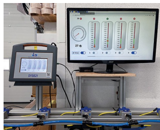
Monitoring system for cleaning nozzles
